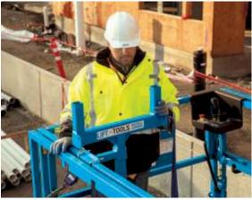
The large carriage and high capacity of the Genie Lift Tools Material Carrier attachment is suitable for multitude of material types, including lumber, pipe, HVAC materials, siding and plate material.
